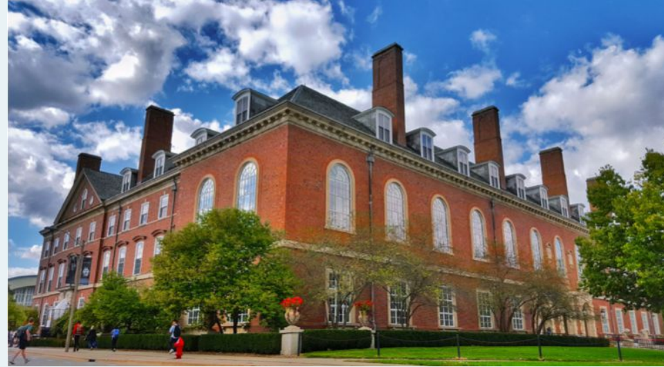
University of Illinois Main Library Building
